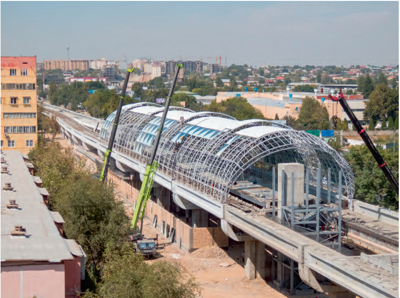
Photo 14.4: Construction of a new station for a surface line of Tashkent Metro along Akhangaran Road
