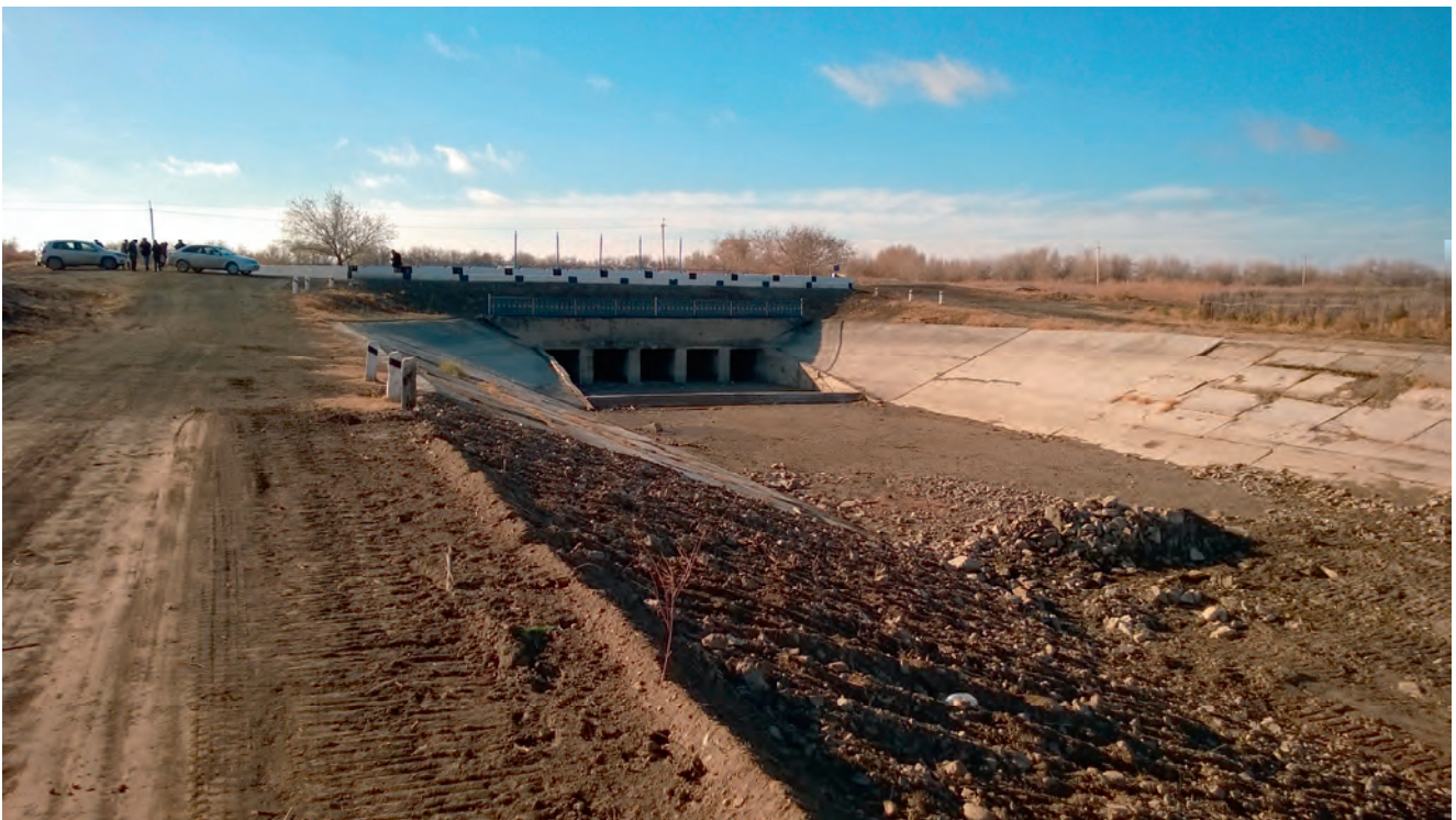
Photo 11.6: Muynak Canal Head at Mezhdurechensk Reservoir
