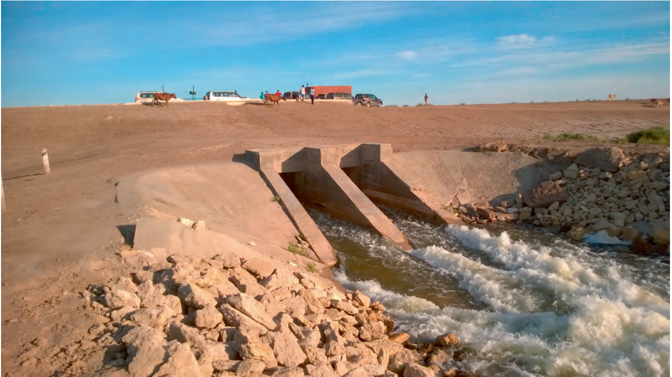
Photo 11.5: Water outlet, Rybachye Reservoir
