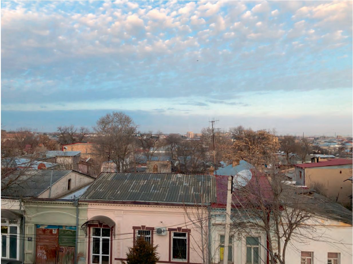
Photo 17: Roofing with corrugated asbestos sheets, Samarkand City
