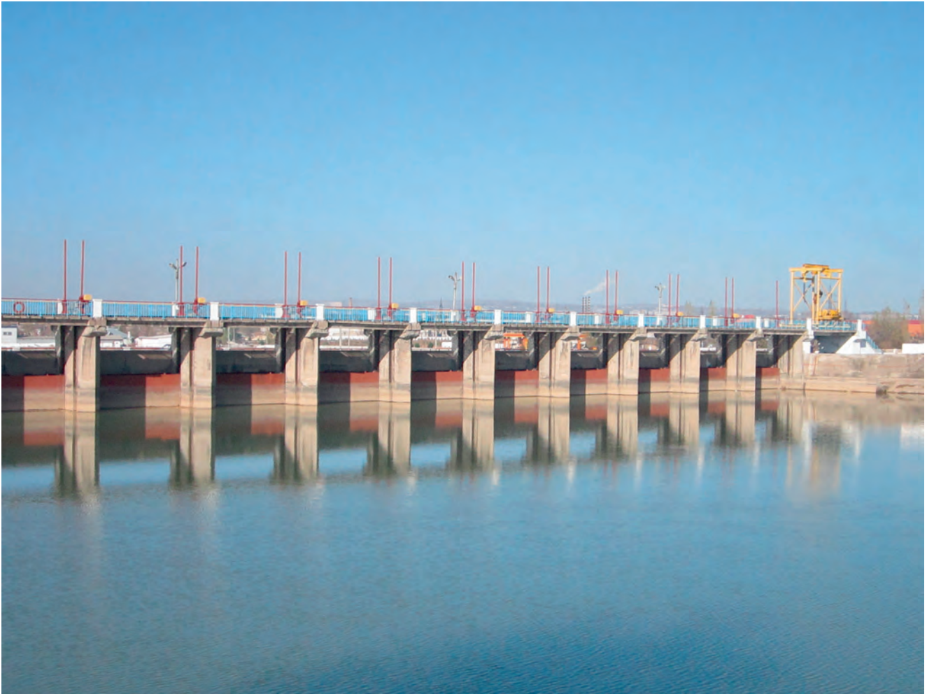
Photo 9.2: Upper Chirchik hydroengineering complex on the Chirchik River
