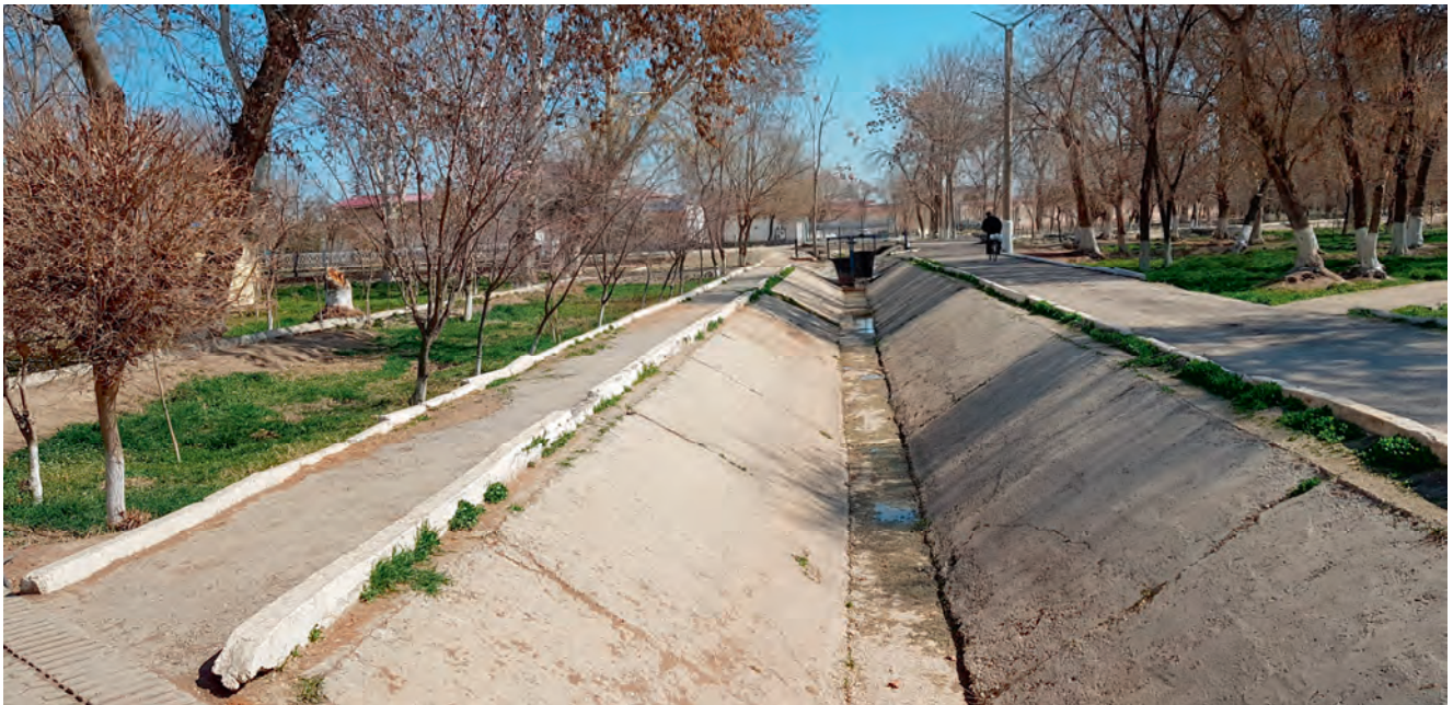
Photo 3: Stormwater channel in Samonids Park, Bukhara City
