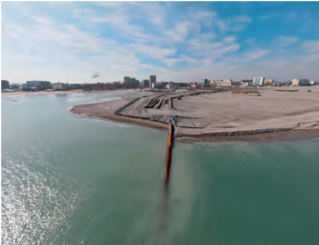
Photo 7.1: Combating coastal erosion, beach reconstruction works
