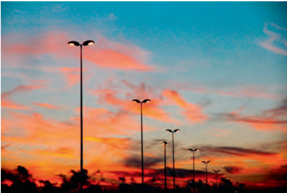
Photo 3.2: Retrofitting old lamp posts with modern remotely-dimmable LED
