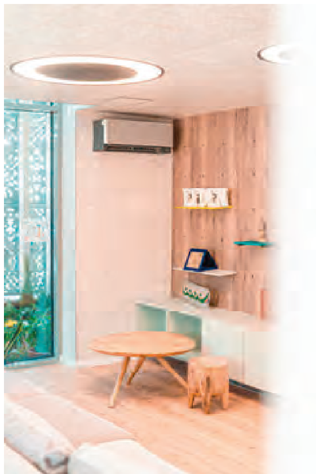
Photo credit: MoEWF, courtesy EFdeN Technical University of Constructions Bucharest
