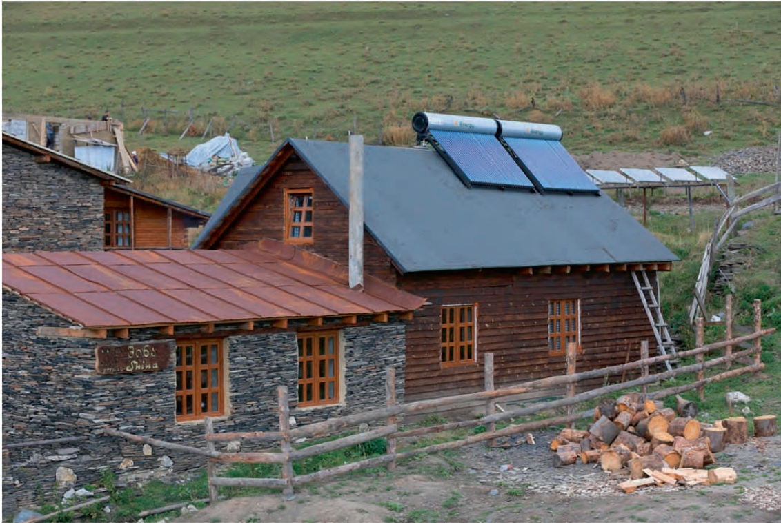
Photo 7.a: Solar panels and solar water heaters installed in Omalo, Tusheti Protected Areas
