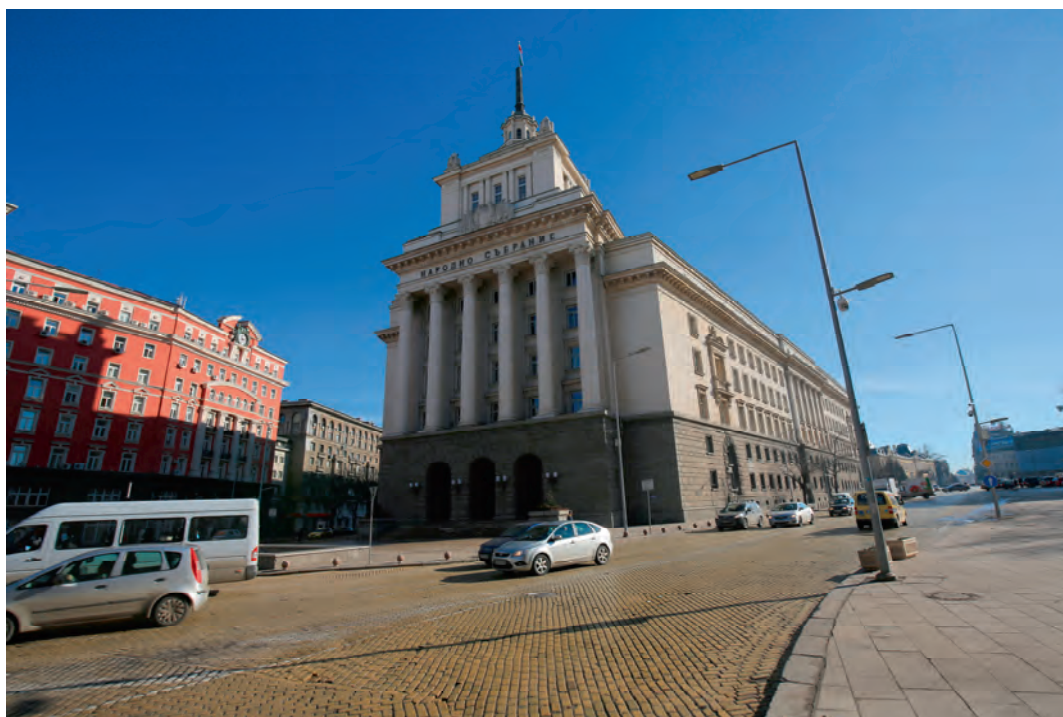
Photo 1: Office house of the National Assembly, Sofia
