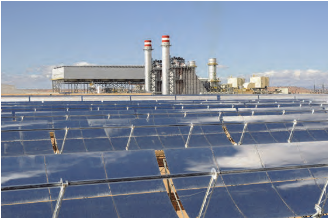
Photo 14.3: Ain Beni Mathar thermo-solar power plant, Oriental region
