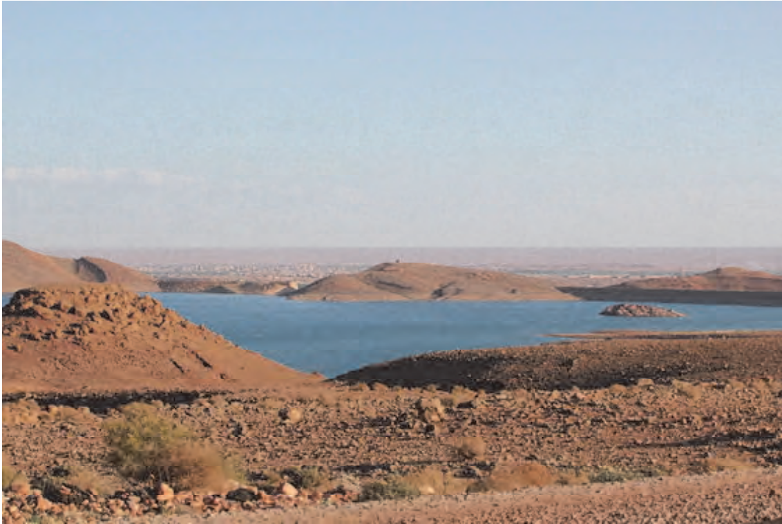
Photo 2.4: Al-Hassan Addakhil Dam
