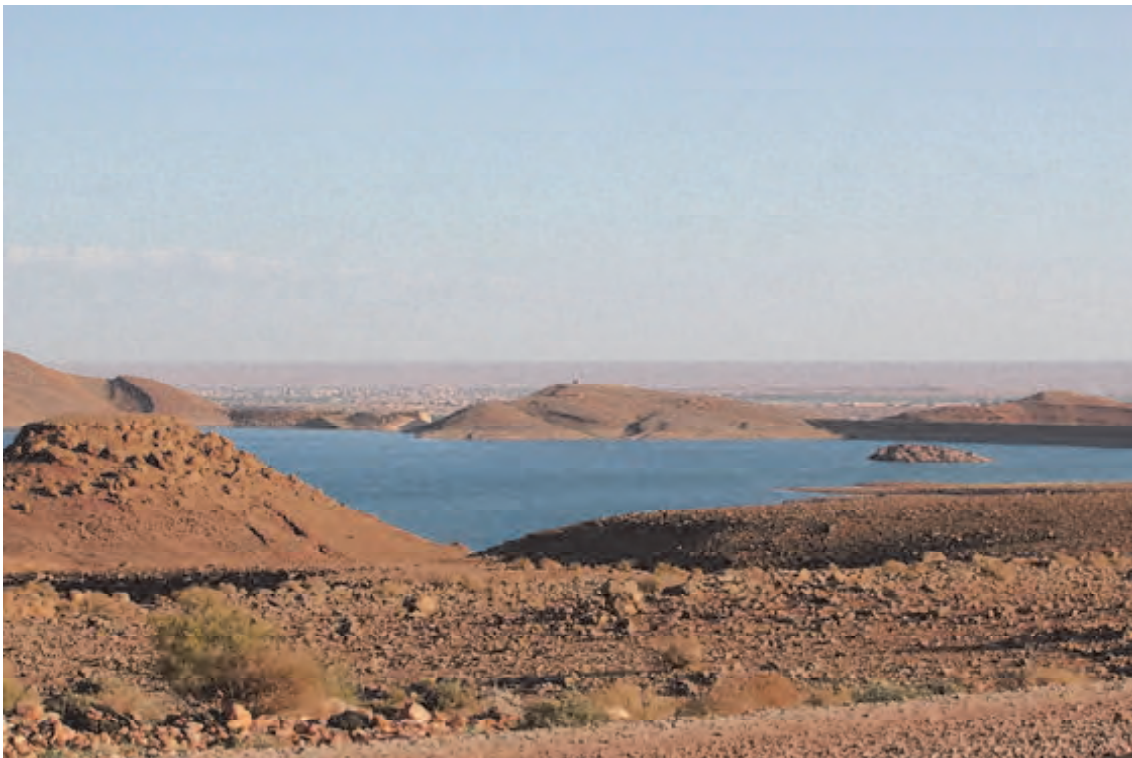
Photo 9.2: Al-Hassan Addakhil Dam
